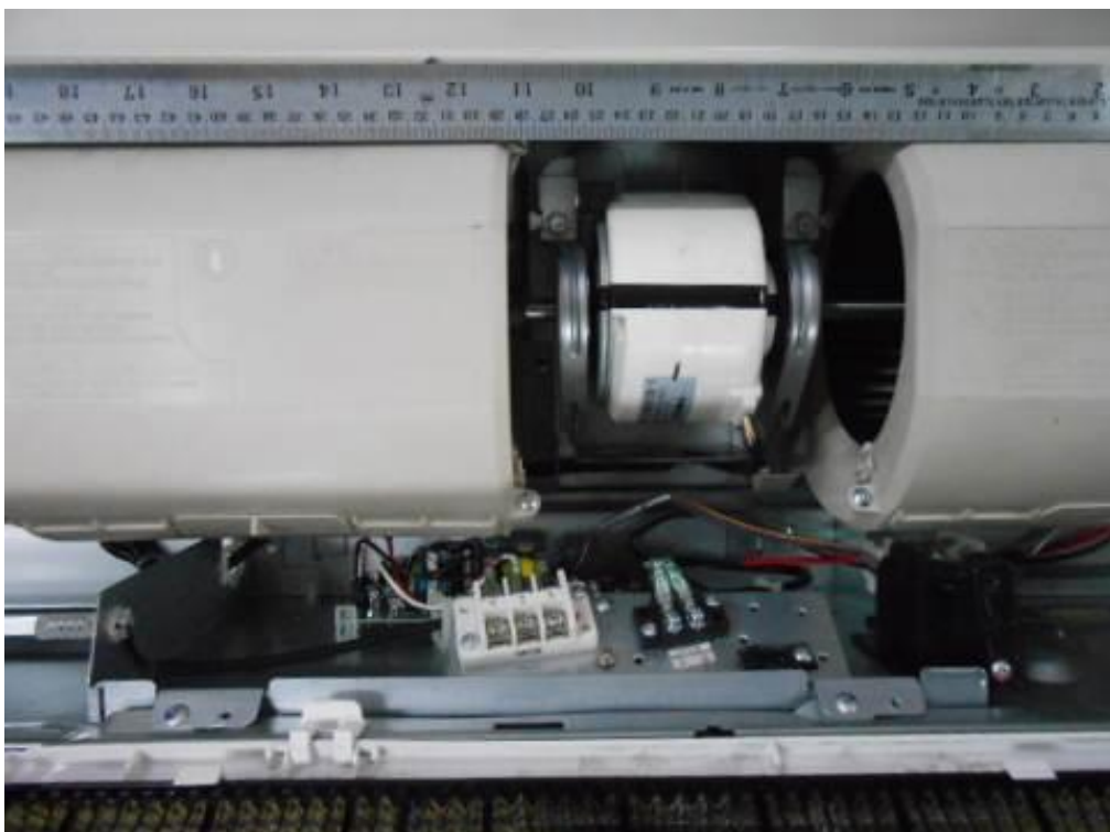
32. RAV-HM1601CTP-E, Fan motor construction of control box. (Representative)
